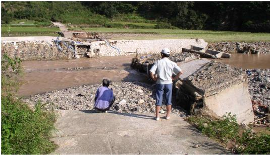
Fig. 1. Bridge loss site due to typhoon Maemi, Sep. 14, 2003.
