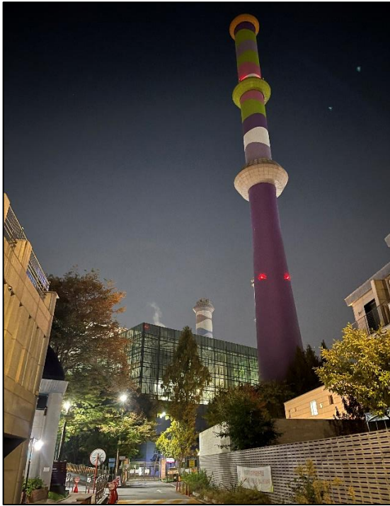
Figure 2: Nowon Resource Recovery Facility
