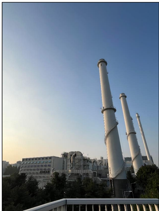
Figure 4: Yangcheon Resource Recovery Facility
