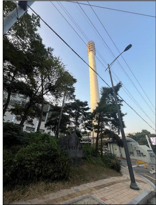
Figure 3: Mapo Resource Recovery Facility
