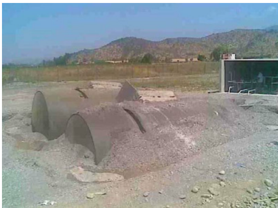
(a) Buried underground tank (Arduino et al., 2010)
