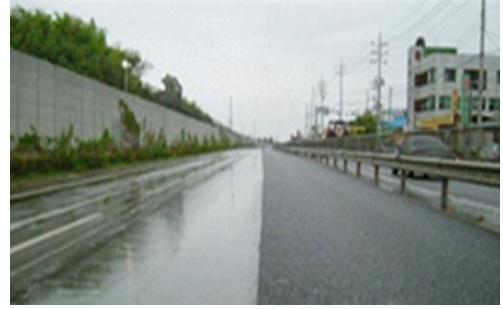
Fig. 7. Comparison of Pavements in Rainy Weather (L: Normal Asphalt Pavement, R: Low-Noise Pavement)
