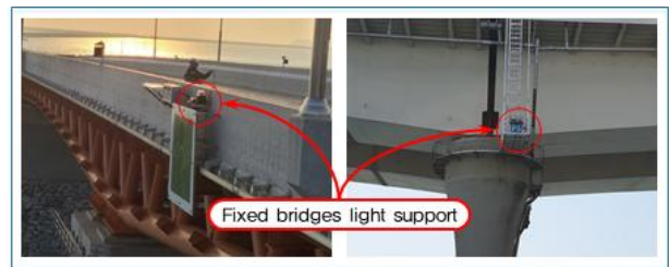
Fig. 3 Example of fixed bridge light support installation
