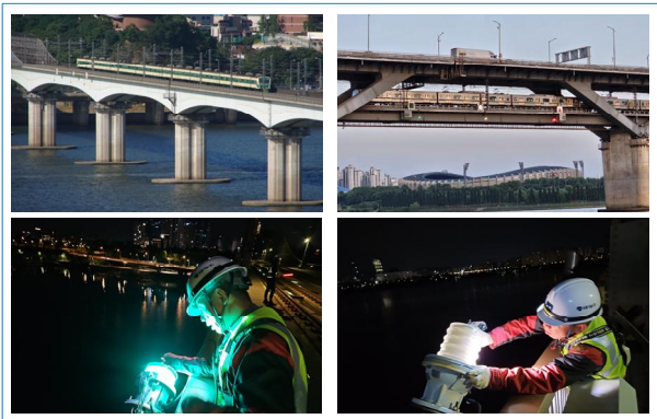
Fig. 6 Example of inspection of railway bridges and bridge lights at dawn
