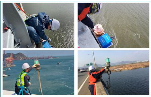
Fig. 5 Example of inspection of bridge lights on marine bridges
