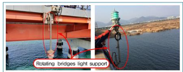
Fig. 4 Example of rotating bridge light support installation
