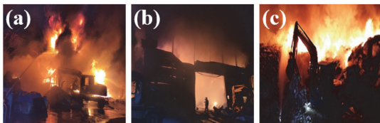
Fig. 2 Example of a fire at a waste facility
