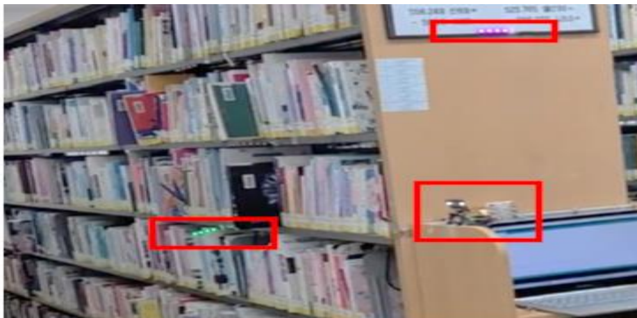
Figure 5. Location notification system installation
