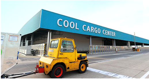
Fig. 7. Cool cargo center at Incheon Airport
