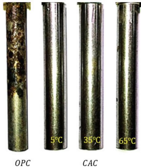
Fig. 4. Visual examination for corrosion of steel in CAC and OPC mortar after the completion of 50 wet and dry cycles depending on the initial curing temperature
