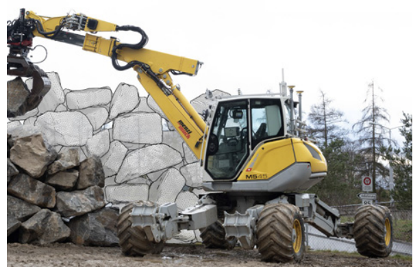
Fig. 8 Autonomous excavator wall construction using digital twin technology 11)
