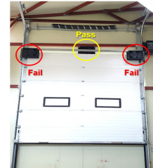
Braking fails(NG) due to balance issues
