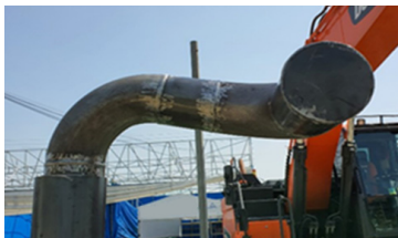
Fig. 7. Test results of self-supporting fall safety device: steel pipe deformation (sag) of 10cm occurred.
