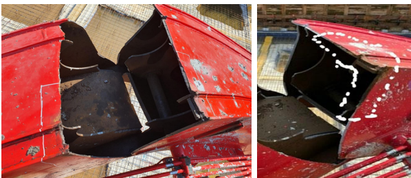
Fig. 4. A sectional photograph of the pump car boom breakage of company D社 (death 2).
