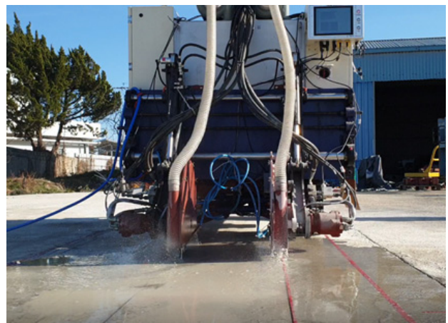
Fig. 8 Driving test of the road cutter
