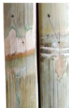
Fig. 6. Drying defects (cracks) during direct drying (a) and indirect drying (b).
