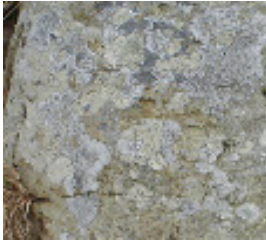
Fig. 11. Drone Photo 1 (angular force)
