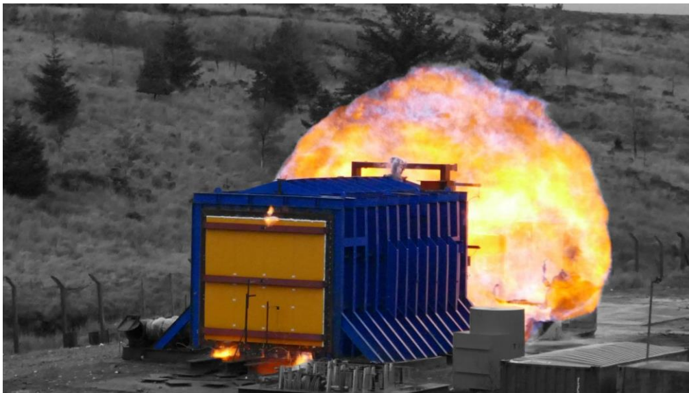
Figure 4. A Facility Designed to Protect the Critical Nodes of Major Crucial Infrastructures
