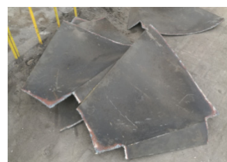
(a) Removal of old blade
