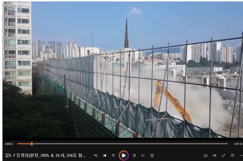
a) dust damage video data at construction
