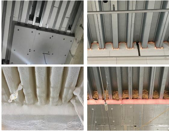
〈Fig. 2〉 Deep-Deck Insulation Construction
