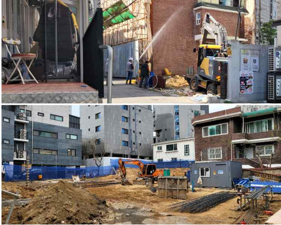
Fig. 1 Usage of excavators at actual construction sites in Seoul
