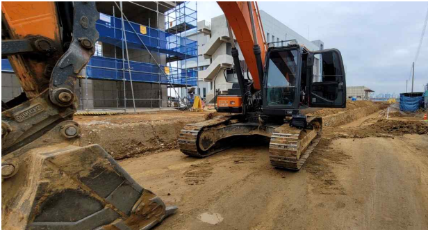
Fig. 2 Excavator used for testing at actual construction site
