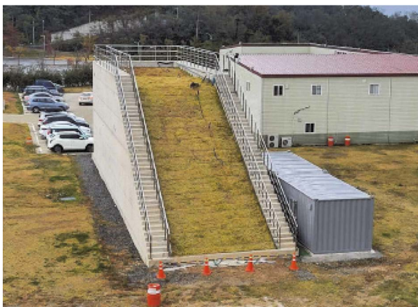
Fig. 6. Panoramic view of the facility.
