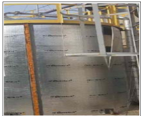
Fig. 1. Accident occurrence facility(Storage Tank).
