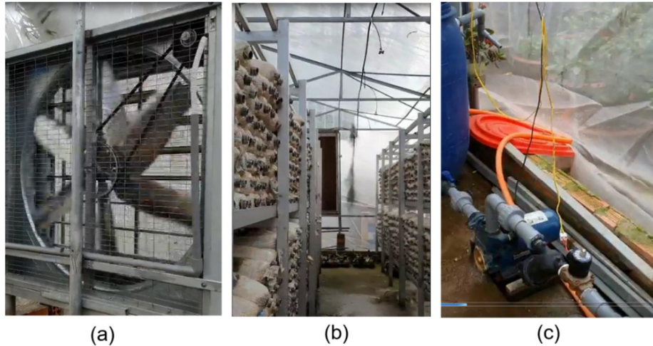
Figure. 2. Components of Control system (a) Fan, (b) Cooling Pad and (c) Pump
