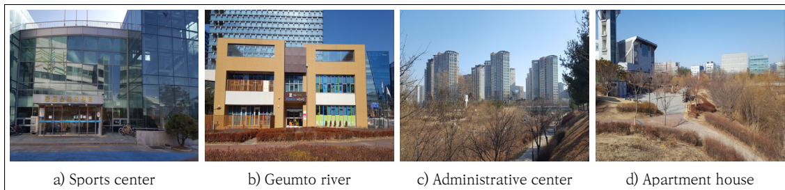
Fig. 4. Status of peripheral facilities.
