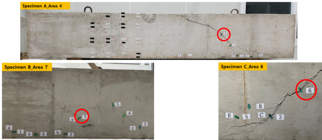
Figure 10. Sensor attachment status for beam member crack monitoring
