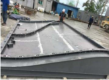
Fig. 2. Formwork for Panels
