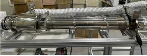
Fig. 7. Duct Type Photocatalyst Filter
