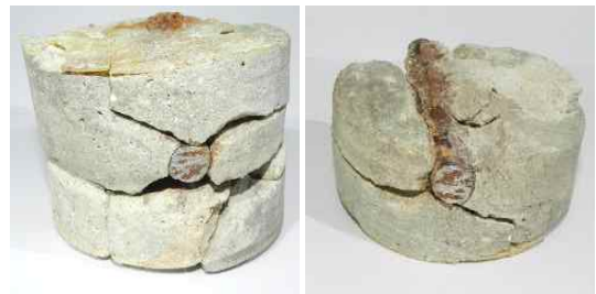
(a) Damaged core (b) Corroded rebar
