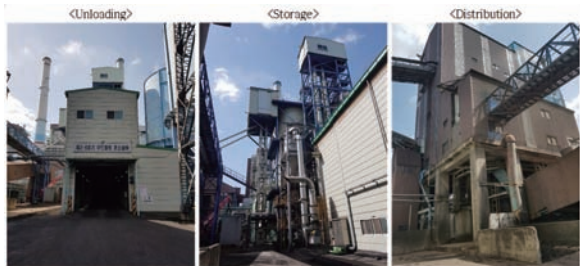
Fig. 4 Biomass mixing facilities of Boryeong power plants
