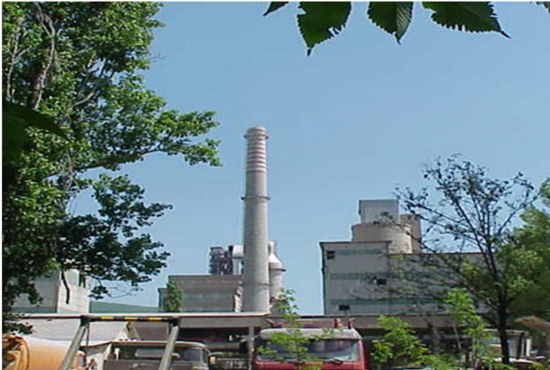
Photo 1. View of the Cement factory chimney
