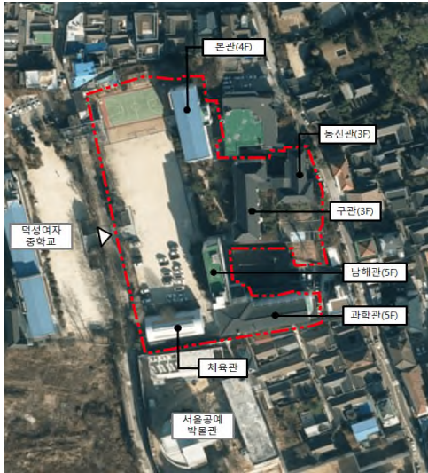
Figure 1. Picture of the current status of D Girls's high school
