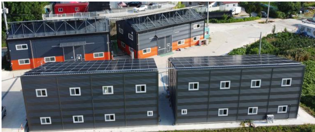
Figure 9. Implementation structure comparison between proposed type (65.4 kW) & conventional A type roof-top plant (78.3 scale)
