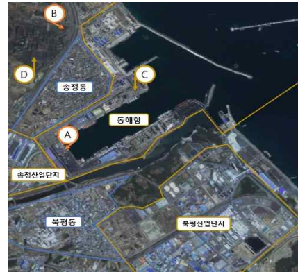
Fig. 2 Residential and industrial infrastructure
