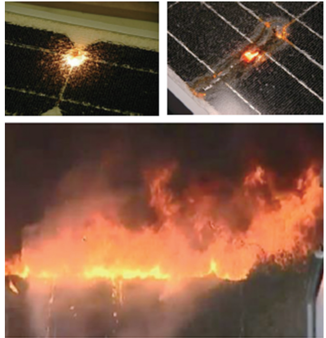
Figure 4. Examples of arc occurring in PV panels (top) and BIPV fires (bottom)
