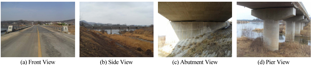
Fig. 5. Target Bridge View
