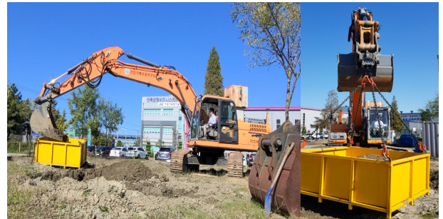
Fig. 3 Weighing test with Hydraulic Excavator
