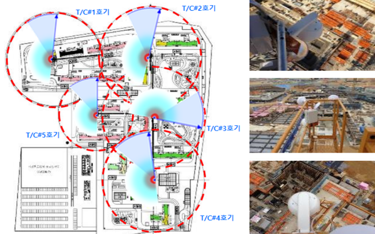
Fig. 2. Wireless CCTV installation
