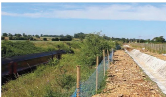
(a) Application of railway lining
