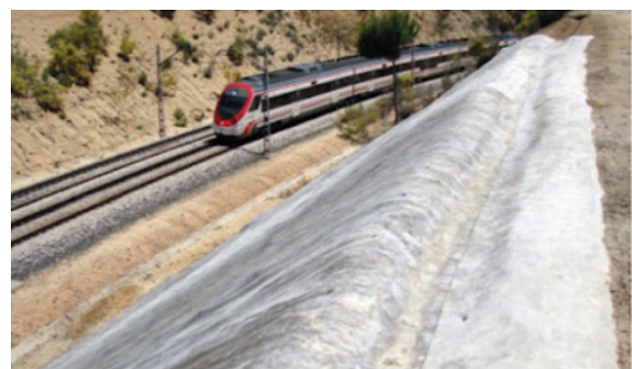
(b) Application of railway slopes
