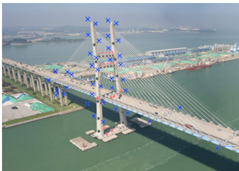
(a) Aerial photograph of Seohae Grand Bridge
