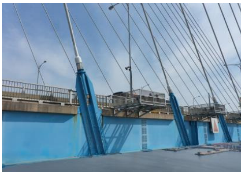
(c) Cable connection part of Seohae Grand Bridge
