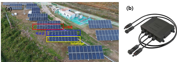
Fig. 1. (a) MW scale PV demonstration site, (b) Prototype PV microconverter
