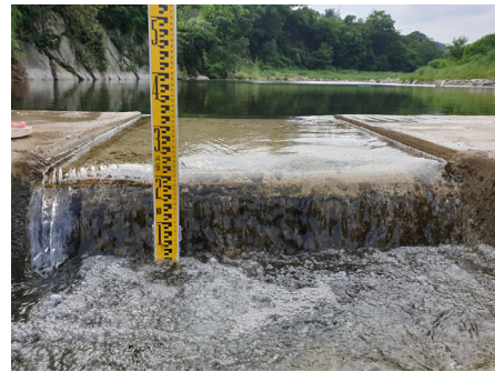
Fig. 4. Critical flow at fishway exit
