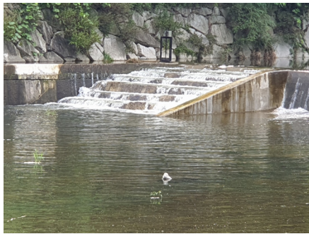
Fig. 3. Stepped boulder fishway installed at Namjeong weir
