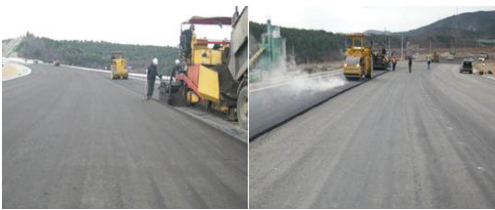
Fig. 2. Road Expansion Work Using Recycled Asphalt
