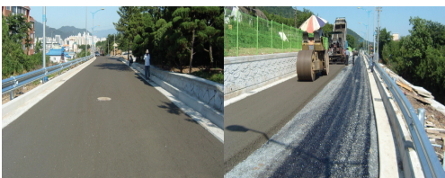
Fig. 3. Road Construction Using Recycled Asphalt
