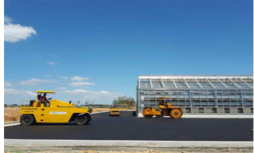
Fig. 4. Incheon Airport 2nd Long-Term Parking Lot Construction Site
