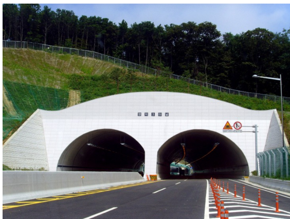
(a) General 2-Arch tunnel
