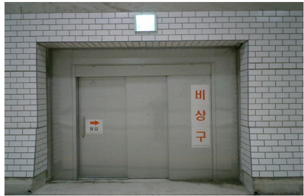
(b) Evacuation passageway in 2-arch tunnel
