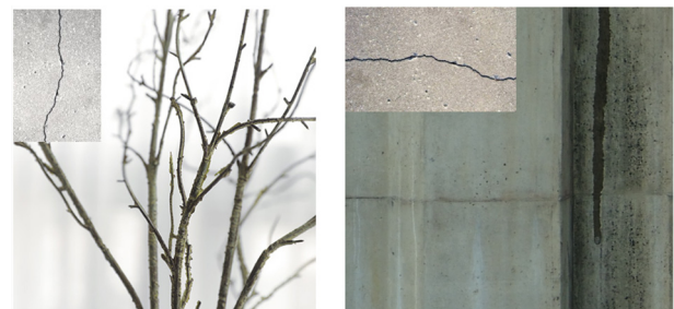
Fig. 3. Examples of hard negative training images (Left: tree branches, right: construction joint).
