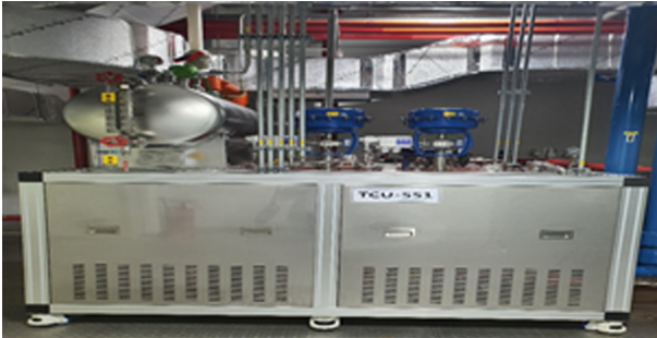
Fig. 10. Backup cooling system in the reaction process.
