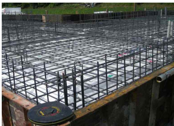
Figure 7. floor rebar reinforcement
