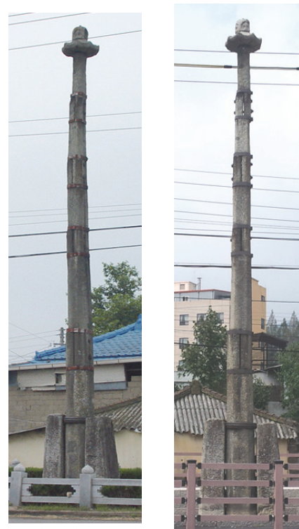
(a) Before restoration (b) After restoration
