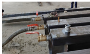
Concrete filled in U-casing
