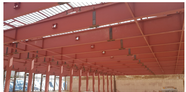
〈Fig. 13〉 Installed TH Beam (Span : 24m)
