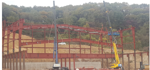
〈Fig. 12〉 TH Beam (Roof) lifting
