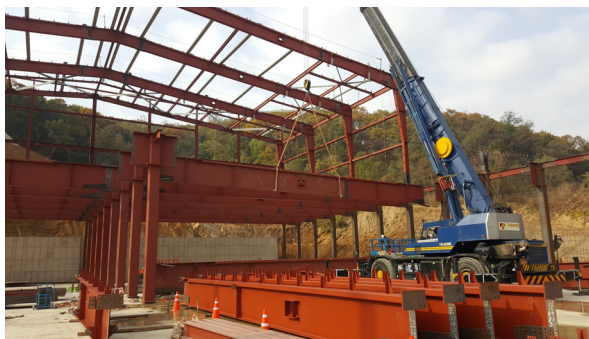
〈Fig. 11〉 TH Beam (2nd Floor) lifting
