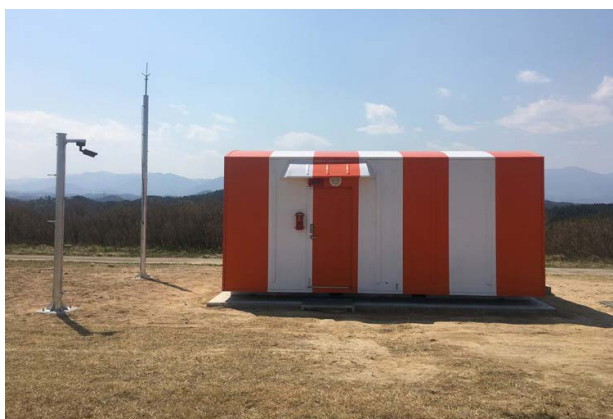
Fig. 3. KRS equipment room.
