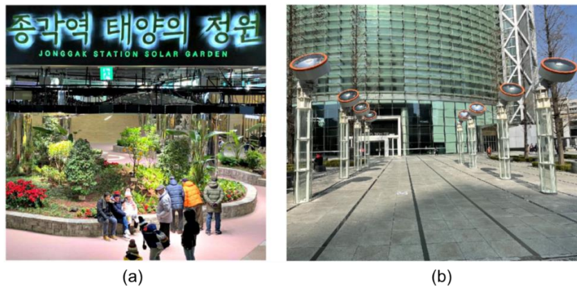
Figure 12. Commercial product of our daylighting system; (a) The system is installed at Jonggak subway station, (b) 8 solar collectors in front of Jongno Tower Square.
