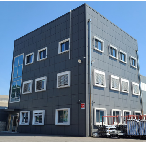
Fig. 1. Building to be Tested
